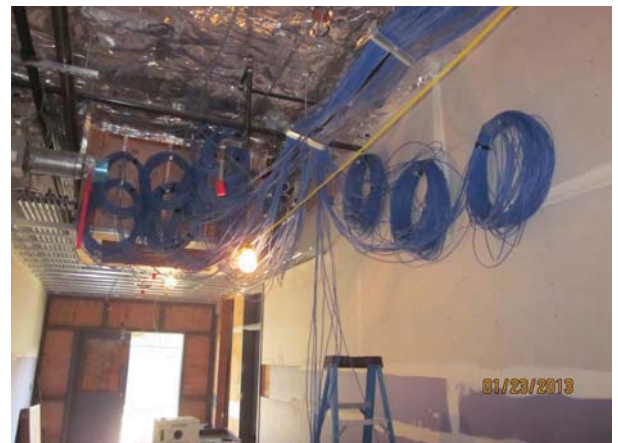
Ductwork in Building A
