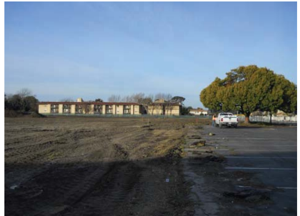
Site clearing and fence demolition
