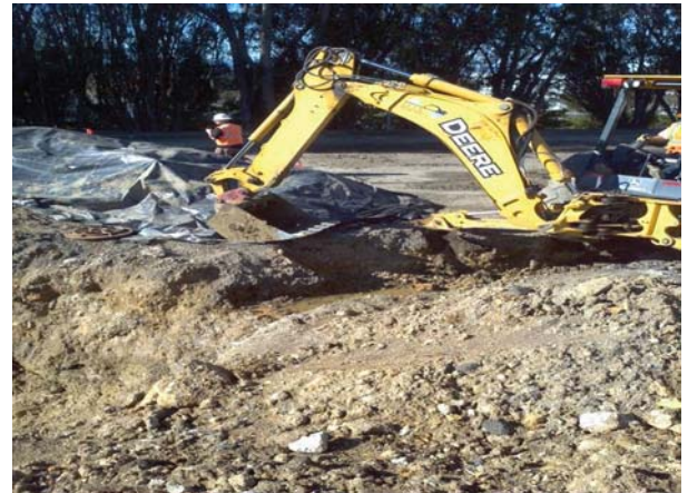
UST Pit additional excavation
