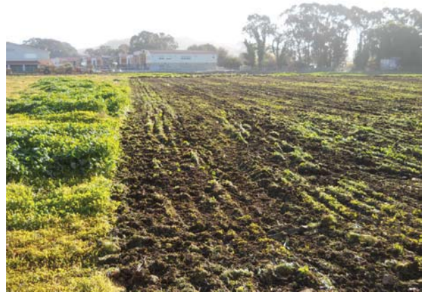
Clearing and Grubbing existing weeds and bushes
