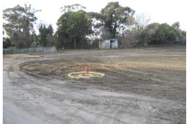
Storm water protection measures installed.
