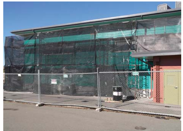
Bldg. E - Installation of Stucco - IN PROGRESS
