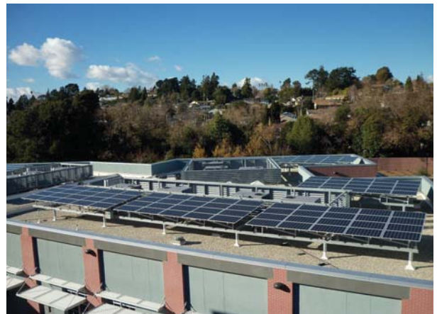
Building No. 3 Roof - PV System Panels
