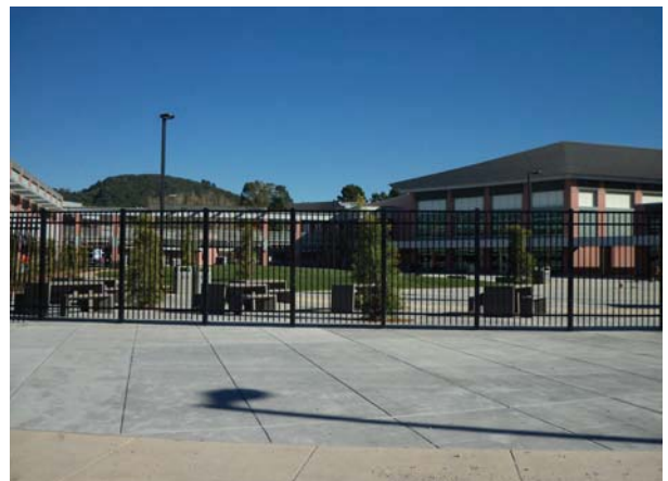
Site Work - Ornamental Fence
