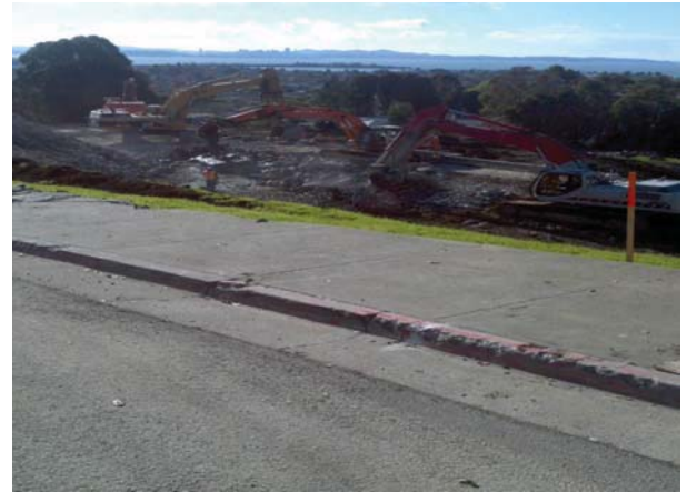
Concrete & rebar removal Main Classroom Building
