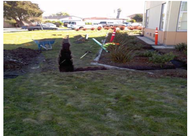
Trenching to existing DI and storm water pipe
