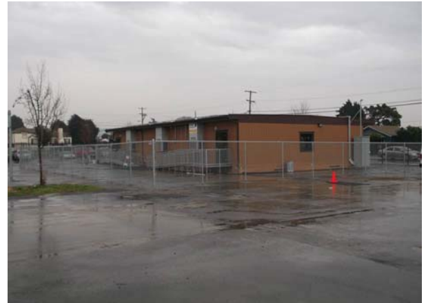
CCS @ Downer Portables, Fencing, Ramps - COMPLETE
