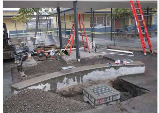
Installation of Underground Storm Drains - IN PROGRESS
