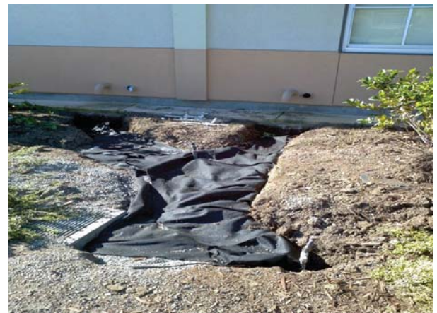
Trench and filter fabric installation at West side of Campus
