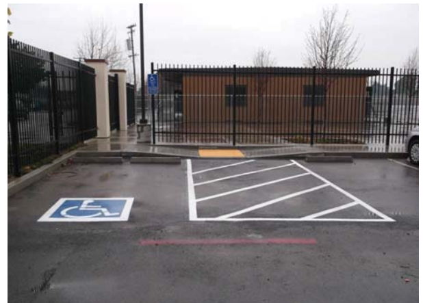
CCS @ Downer- ADA Parking & Gate Opening - COMPLETE
