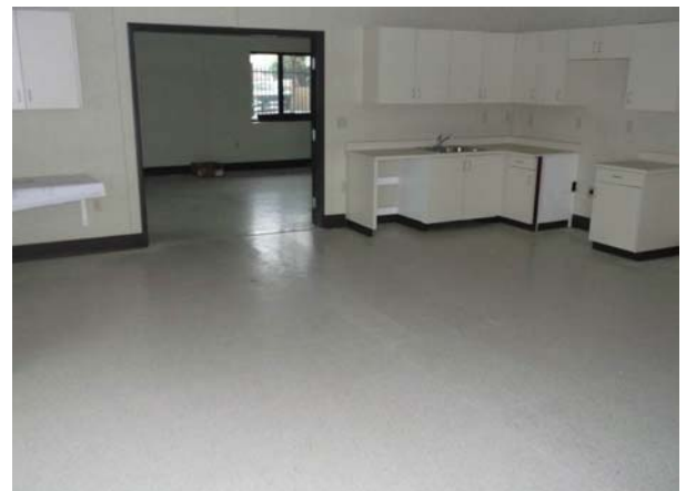
CCS @ Downer-Cabinet Installation - COMPLETE
