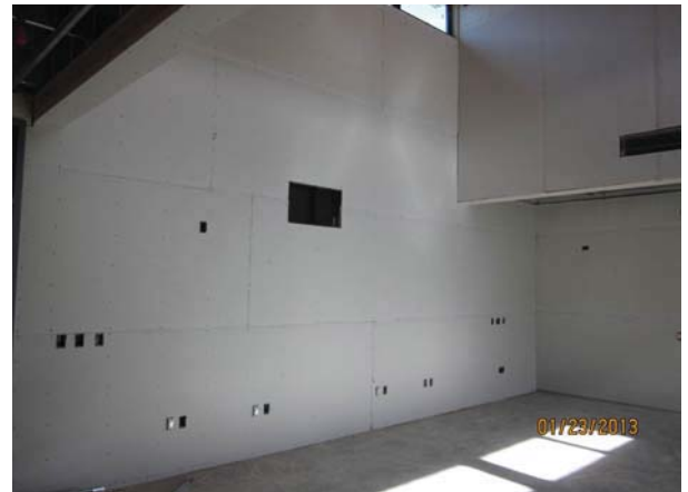
Clerestory Window Installation on Building B
